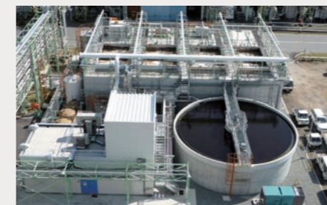
Activated sludge treatment facility prevents sea and river pollution by detoxification of factory effluents.
