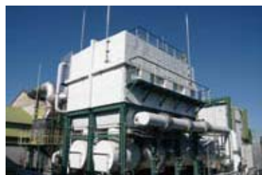
Incineration unit to treat exhaust gases from the synthetic rubber drying process
