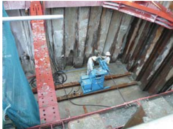
Soil improvement work to improve earthquake resistance (Chiba Plant, JSR Corporation)
