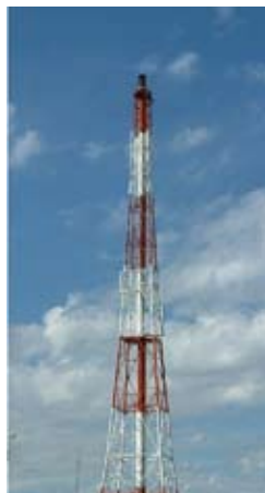
Waste gas from the plant is incinerated in a flare stack
