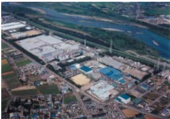
Toray Industries, Inc. Gifu Plant
