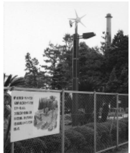
Installation of street lights by solar and wind power generation
